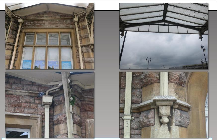
Pigeons had been roosting and nesting for many years below the glass canopy on the upper horizontal ledges (top left), the inside of the canopy frame (top right), the hoppers and drainpipes (above left) and the thrush bearings which support the arched metalwork (above right). This necessitated frequent cleaning of pigeon droppings from the pavement below the glass canopy.
